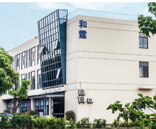
JANDC Co., LTD. headquarter in Kanagawa, Japan.
